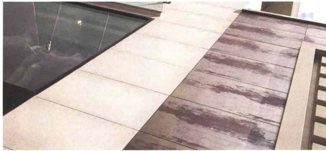
▪ The facade in the photo (designed by Gino and Emiliana Pisoni) was built with ceramic tiles from the Active collection, which interacts with the environment to reduce pollutants by up to 70% thanks to the presence of titanium oxide particles on the surface.
